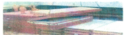
Remark: WELDED FLAT BARS ON SIDES DETACHED
